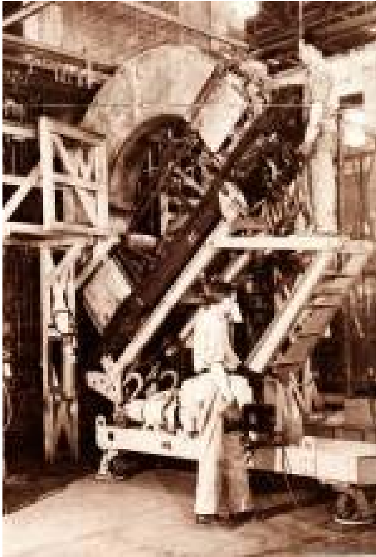
Figure 5-2. Calutron Unit
