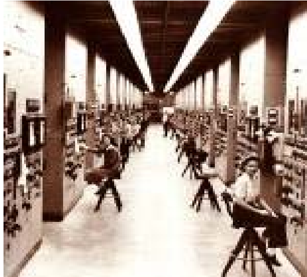
Figure 5-7. Control Panels and Operators for Calutrons at Oak Ridge. The Operators, Mostly Women, Worked in Shifts Covering 24 Hours a Day
