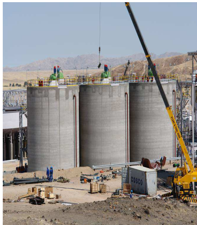
FIG. 7. Leach tanks during construction.
