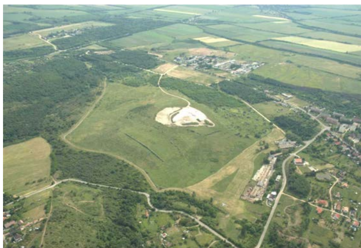
FIG. 4. The remediated waste rock pile N3. On the top the still operating storage area (for water treatment sludge) can be seen.
