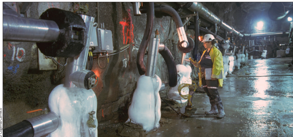
Raise boring in frozen ground in the McArthur mine (Canada).
