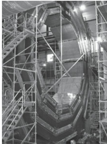
[ FIGURE 38 ] CMS's magnetic return coil interlaced with its muon detector—all under construction.
