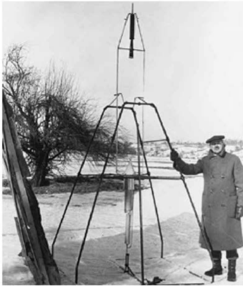
Goddard standing next to the rocket that made history on March 16, 1926, when it became the first to fly with liquid fuel. The rocket itself is the dark machine at the top of the frame. (NASA)
