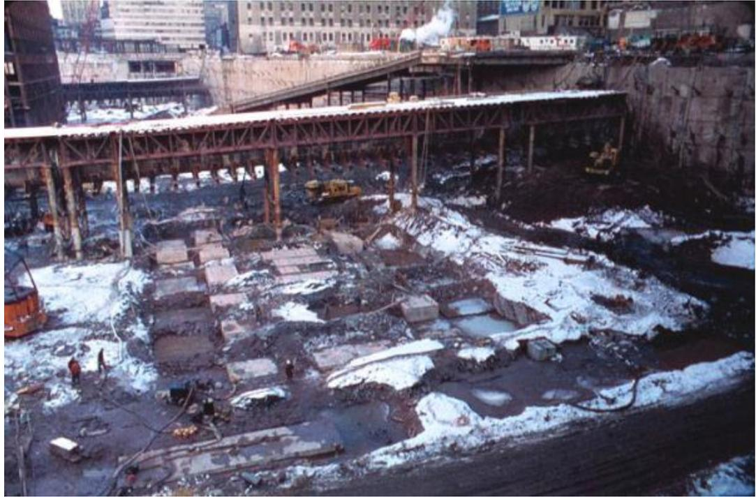
This construction photograph shows the foundation of South Tower in the foreground, with the foundation of the North Tower in the left background. The foundations were seven stories deep.
