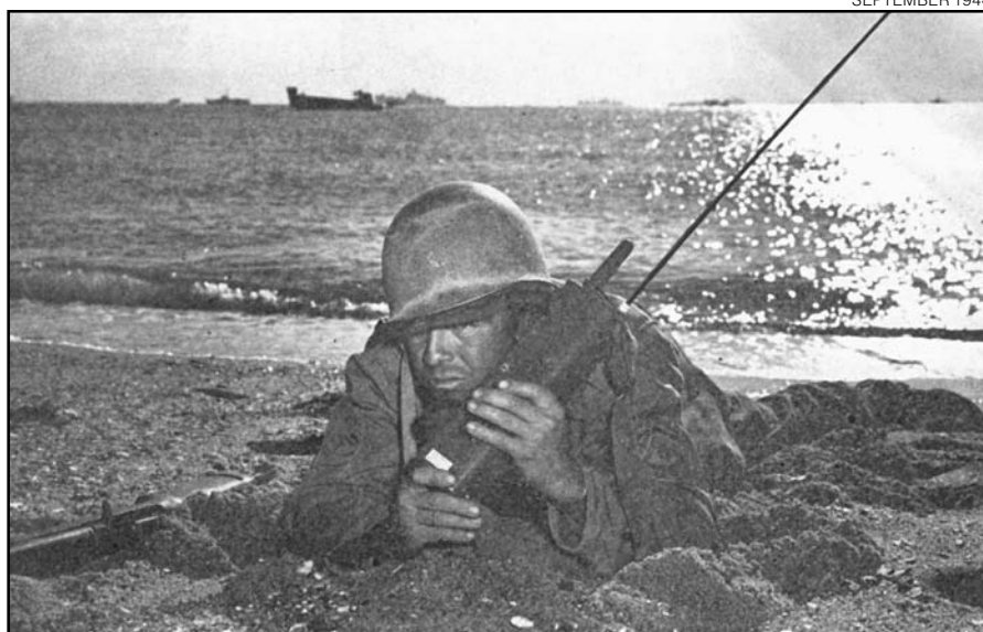
Figure 5—From an article on the Signal Corps, a photo of a sergeant using the Motorola SCR-536 Handie-Talkie in field conditions during a military training exercise.
